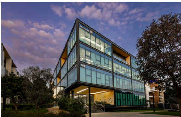
NFO Johannesburg Offices
